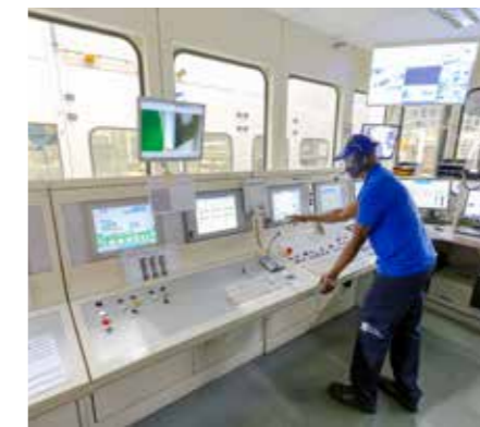
In de controlekamer
